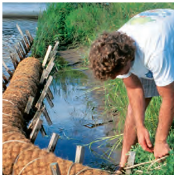
Fiber logs are one option for stabilizing the shore.
